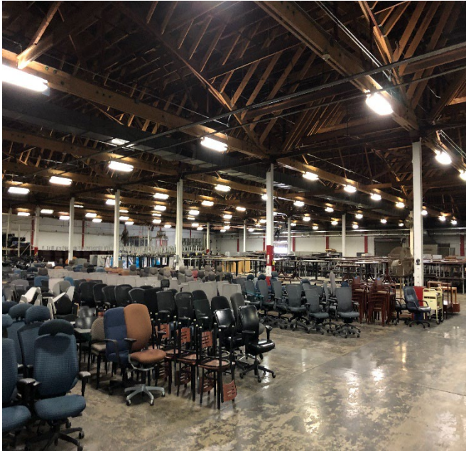
Image 1 - Floor storage for larger items
